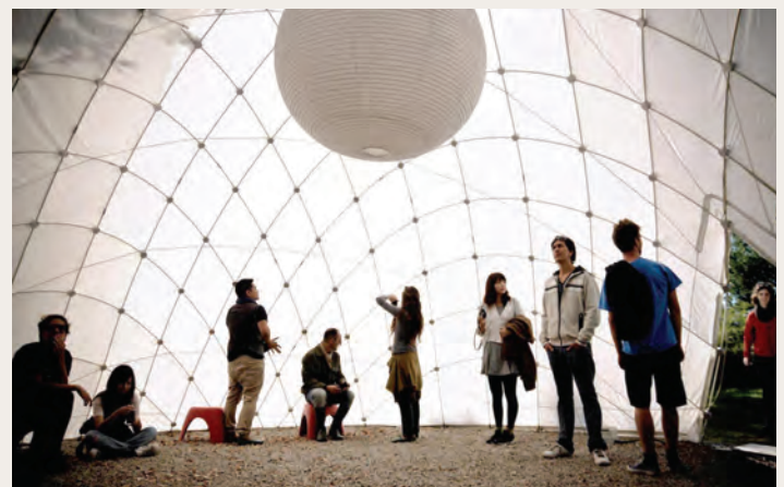
Jorg Schlaich <The Bamboo-and the Fibreglass-Dome> 2009 Fibreglass rods connected with specially manufactured aluminium sleeves and spanned with a tear-resistant, weatherproof and translucent membrane © Domaine de boisbuche
